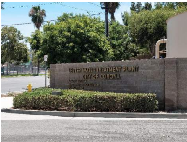
Figure 5 LESTER WATER TREATMENT PLANT
